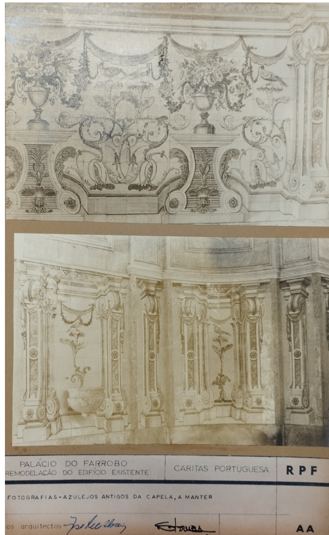
Figure 10 - Photographs of the old tiles from the chapel of the Farrobo Palace, (AHVFX, Urbanization Studies Office, application 02332, 23 July 1970, Farrobo Palace remodeling process).
