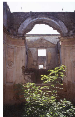
Figure 7 - An aspect of the ruined interior of the Farrobo Palace chapel, Vila Franca de Xira. Unknown, 1982, Col. Municipal Museum of Vila Franca de Xira.
