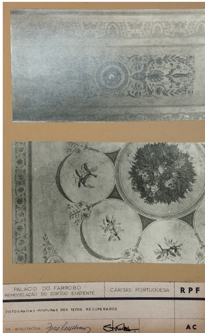
Figure 13 - Photographs of the old wall paintings of the Farrobo Palace, (AHVFX, Urbanization Studies Office, application 02332, 23 July 1970, Farrobo Palace remodeling process).
