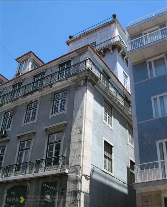
Figure 9 – Buildings on Rua do Alecrim, nº 38 to 54, Main facades, right side and observation deck (South building), photography by Inês Pais, 2006, (SIPA, PHOTO.00808817).
