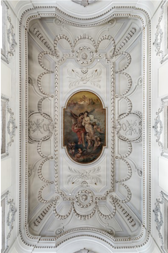
Figure 12 - Palácio das Laranjeiras, ceiling of the staircase house, João Paulo da Silva (attribution). The composition of this ceiling, still with quadratures marking the four oblique panels, and cartouches with shells, takes us back to the late-Baroque or Rococo period. However, the relief stucco ornaments, which extend to the overdoors, are already of a neoclassical taste: the heavy garlands and festoons of laurel leaves, the logs of oak leaves, the quill feathers tied with bows and the lion's heads.
