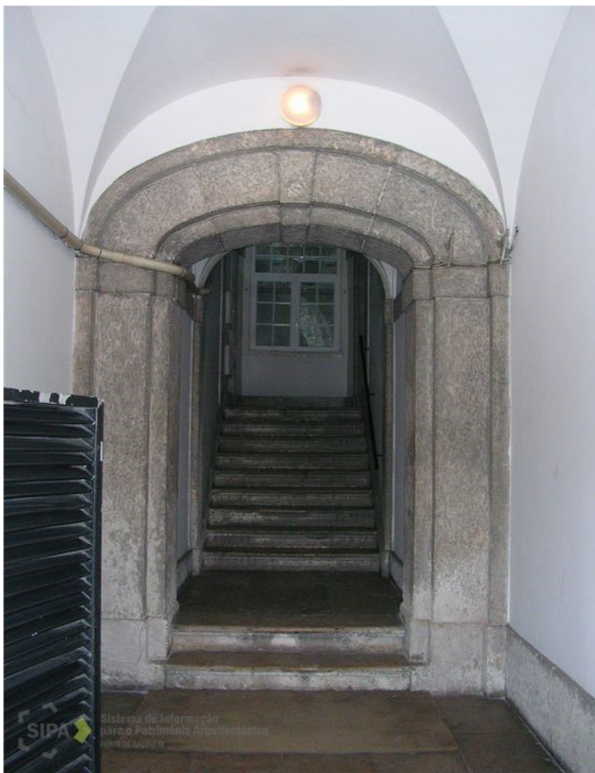
Figure 7 - Buildings on Rua do Alecrim, no. 38 to 54 - Interior: atrium (South building), photography by Inês Pais, 2006, SIPA, PHOTO.00808814.
