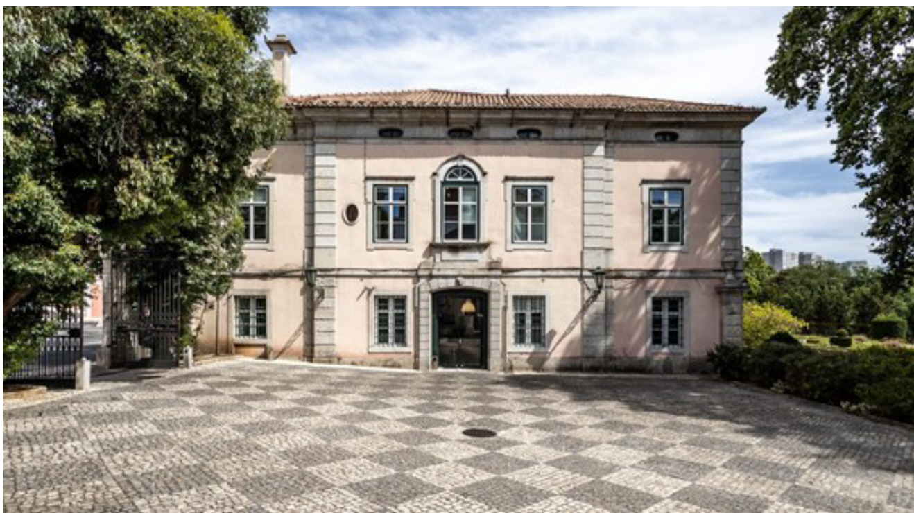
Figure 6 – Façade of Quinta das Laranjeiras over the receiving yard, photograph by José Vicente, 2023.
