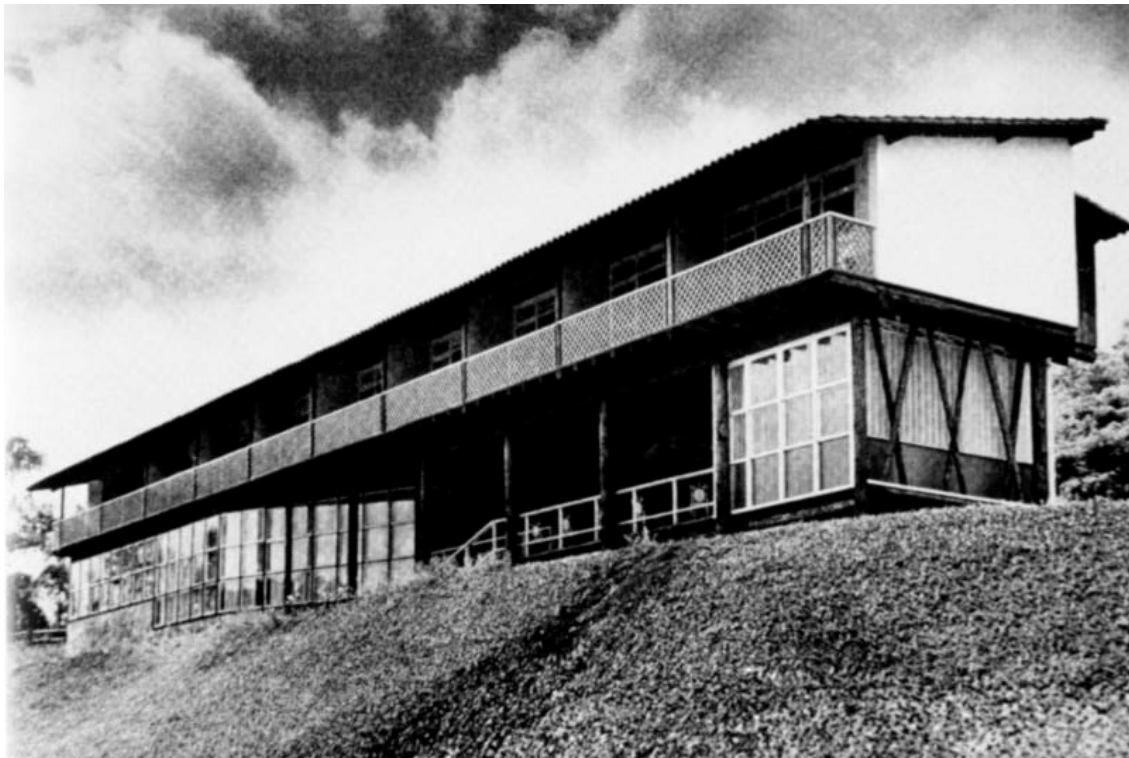
Figure 4. Park-Hotel São Clemente, by Lúcio Costa, express his ideas about the synthesis between modernity and tradition, the main feature of the Brazilian modern architecture (Source: Wisnik, 2001)
