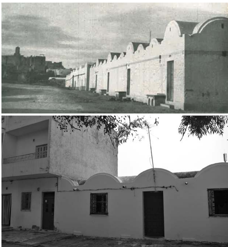
Figure 3. Sousse, Tunisia (1948, 2014). The housing complex in Sousse is an example of the "maison minimum" being applied. Built by the architects Lu Van Nieuw and Greco, transformed without an architectural logic to respond to growth and to the needs present, by raising and distorting the original matrix.
