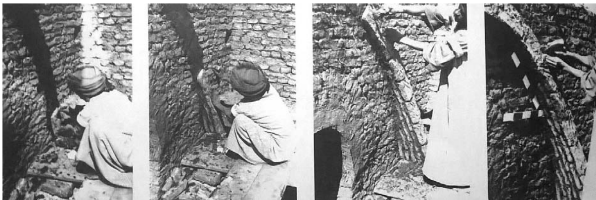
Figure 1. Mude domes being built (Fathy, 2009 [1969]: 22).
