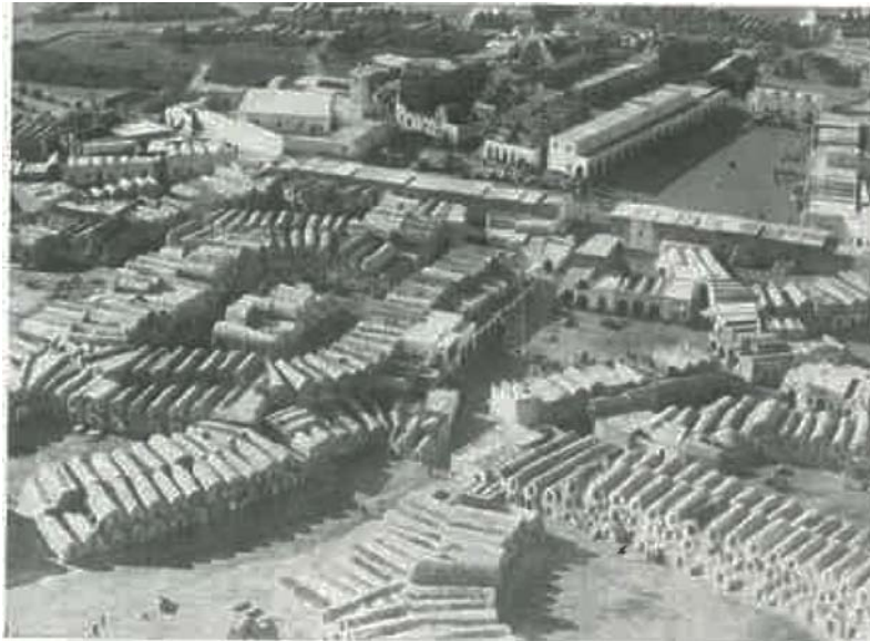
Figure 1. Medenine, Tunisia. Located at the crossroads between Djerba, Libya and South Sahara, has been a capital since the sixteenth century. It was the meeting point of the nomadic community. Here had concentrated the fortified granaries, which represented a strategic point for the Tunisian territory. The form of a huge "Ksar", and the minimalist home are examples of typical rational construction.
