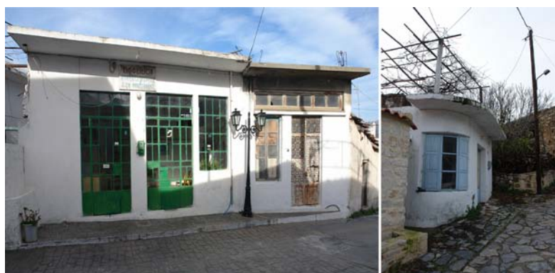
Figure 2. Typical buildings on the main streets of the villages of Aghios Georgios (Lassithi Prefecture) and Mourtzaná (Rethymno Prefecture) in Crete. Photographs by the author.
