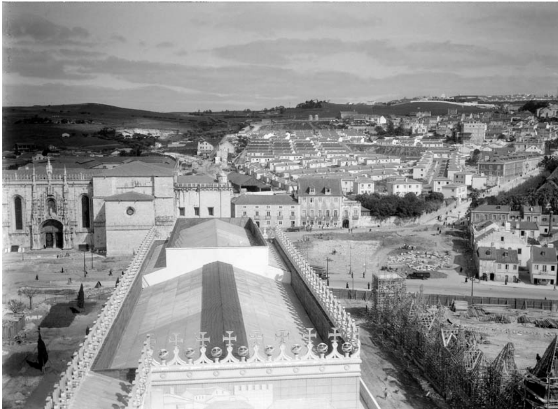
Figure 4. The Affordable Houses Neighbourhood of Belém behind the Monastery of Jeronimos, Lisbon, in 1938-39. Construction works for the Portuguese World Exhibition of 1940 are visible on the bottom right (source: Biblioteca de Arte, Fundação Calouste Gulbenkian).
