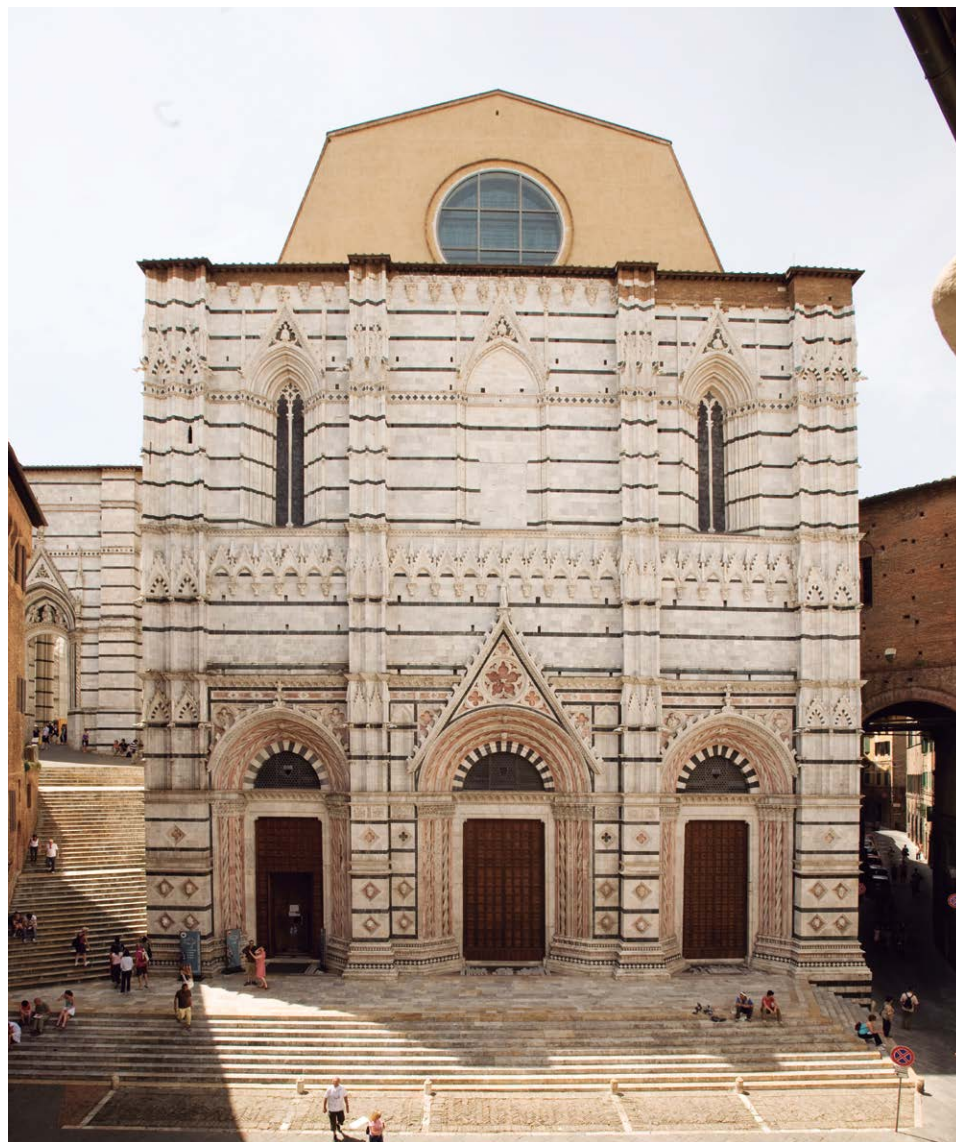
Fig. 3 - The rear façade of the cathedral.
