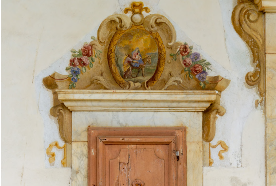
Fig. 7 – Painting on the top of the small door used to bring food to the monks, preserving their isolation (north arm, “P” cell). Differences in colour and grain are visible between the paint closest plaster and the surrounding portion (photo by the authors, March 2019).
