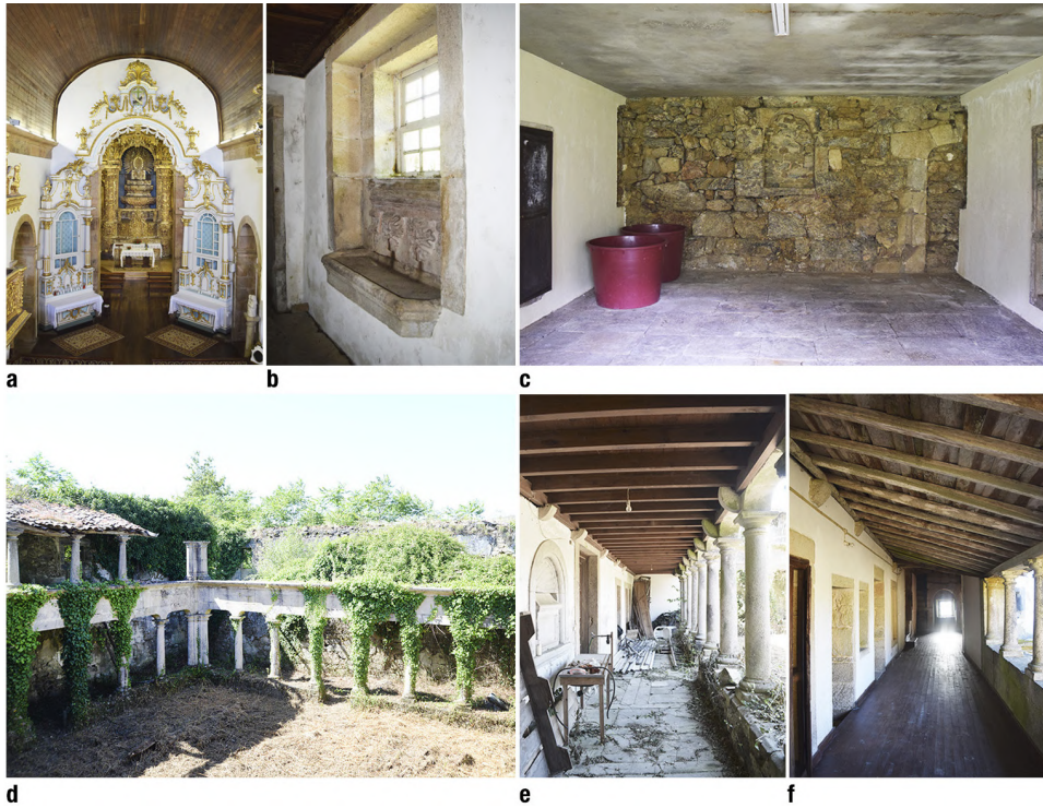
Fig. 6 – Photographic survey: church's nave (a), lavatory house (b), sacristy (c), cloister (d), confessional corridor (e), and choir corridor (f). ©Rolando Volzone, 2021.
