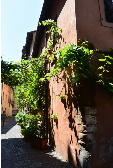
Fig. 2 – Rome, via in Piscinula. Church of St. Benedict in Piscinula, the left corner with traces of pre-existing buildings. ©Maria Grazia Turco, 2018.
