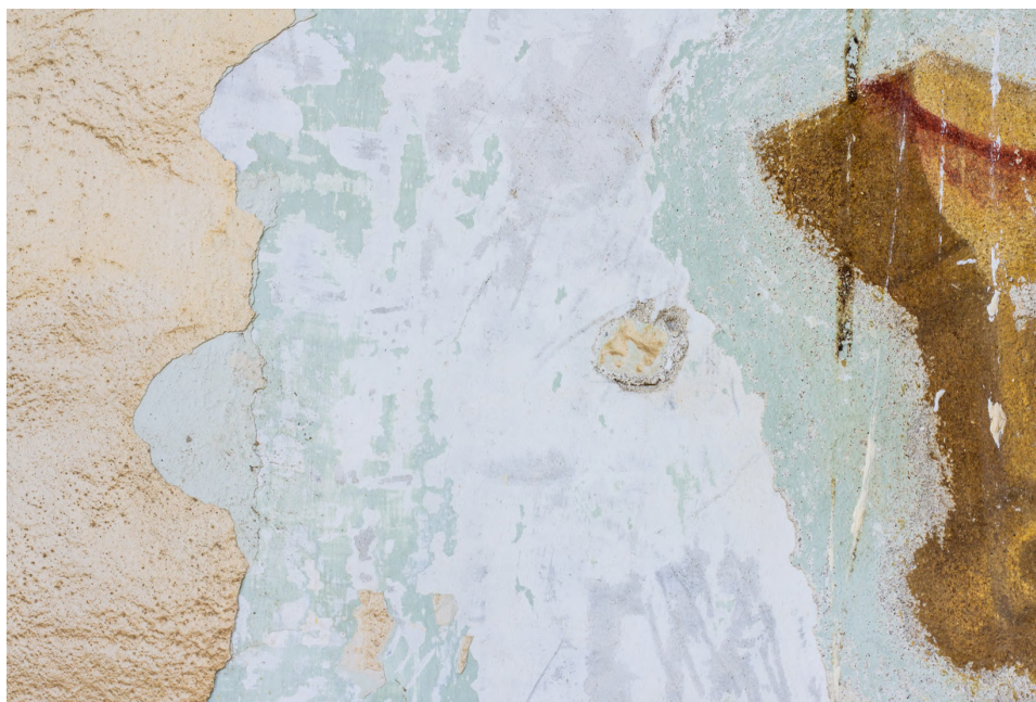
Fig. 4 – Traces of two different green paint layers under a yellow one in the east arm (photo by the authors, October 2019).
