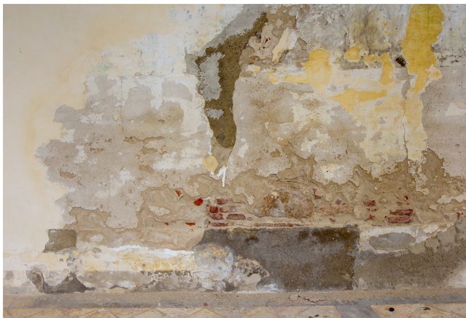
Fig. 6 – Portion of north interior façade where traces of the newest white paint layer, the yellow and the green ones are visible. On the bottom there are two different treatments of the grey strip: on the left there are traces probably of the newest, which is thinner and lighter in tone than the older in the middle of the photo (photo by the authors, March 2019).
