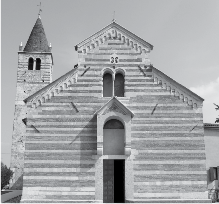
Fig. 7 – Belfiore (Vr), San Michele: facade of the church. Photograph by the author.
