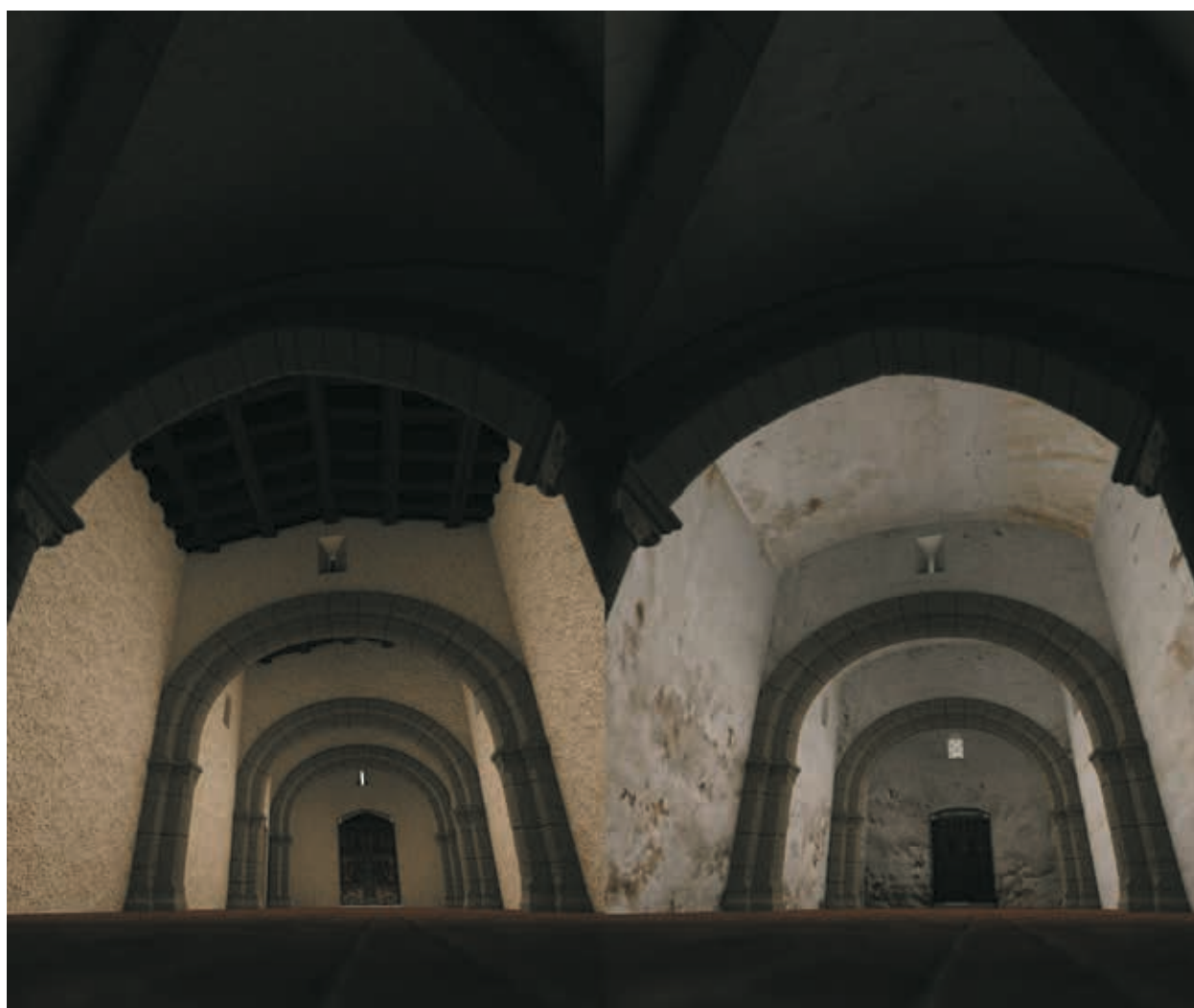
8. Interior view of the changes between the 3 rd (left) and the 4 th (right) phase, with the implementation of the vault roof in substitution of the wooden roof and the drawback of the facade on the right interior view with the elimination of one of the arches.
