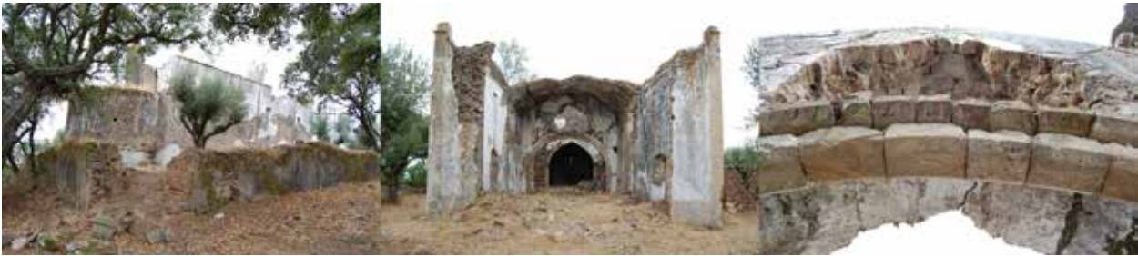
1. Current state of the ruin of the hermitage church of Santo André do Outeiro.
