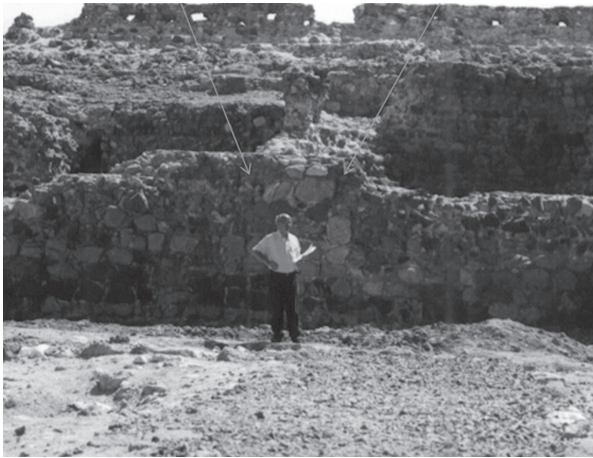
12. Face interior do "baluarte semi-poligonal" (2001).
